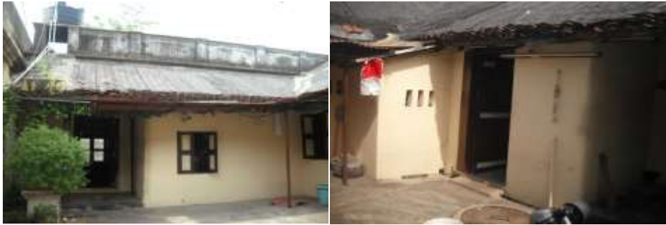
Fig 11. View of Thulasi madam in the courtyard and view of courtyard form the kitchen
