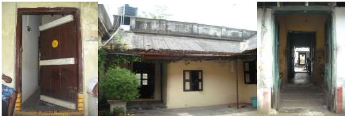
Fig 9. Doors and windows with a yellow paint where turmeric is used for hygiene. Staircase with lime concrete and Thulasi madam with a courtyard can be seen
