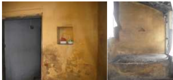
Fig 7. Pirai as a traditional design feature in traditional houses - cuboidal and prismatic recess
